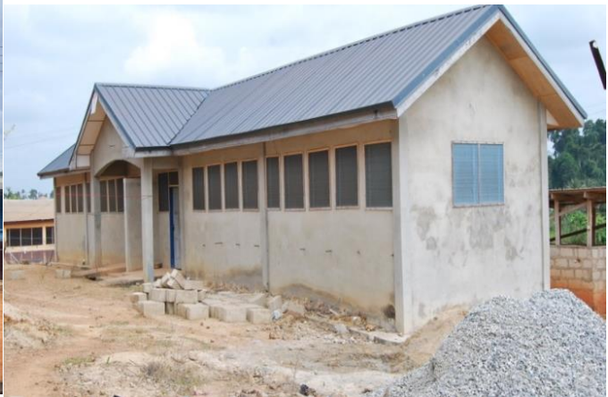
Boys Latrine at Nsaba SHS
