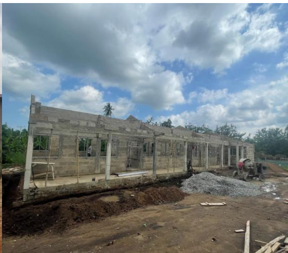
Ongoing construction of 3-unit classroom Block at Agona Nkumkum (35% completed)
