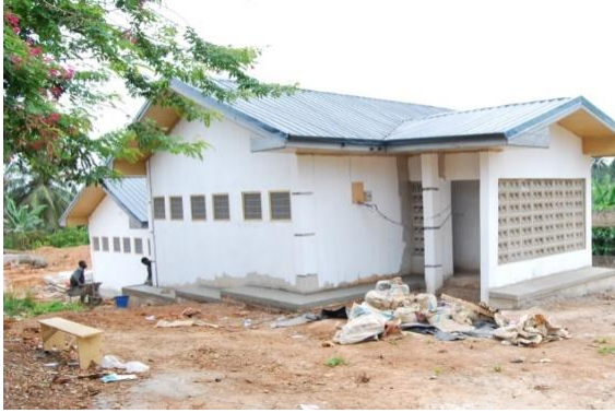
Girls Latrine at Nsaba SHS
