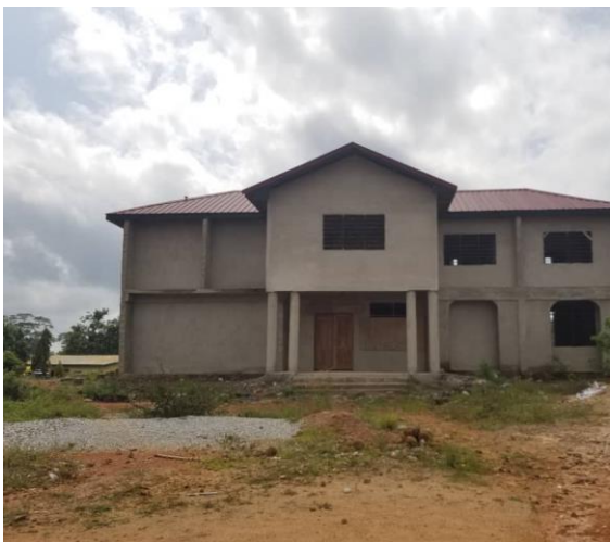
Police Station at Agona Nsaba (80% completed)
