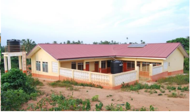
New Kindergarten block at Kokoado
