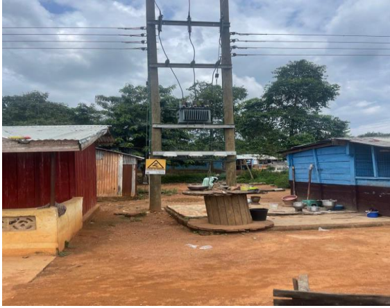
Extension of Electricity to New Communities in Duakwa.
