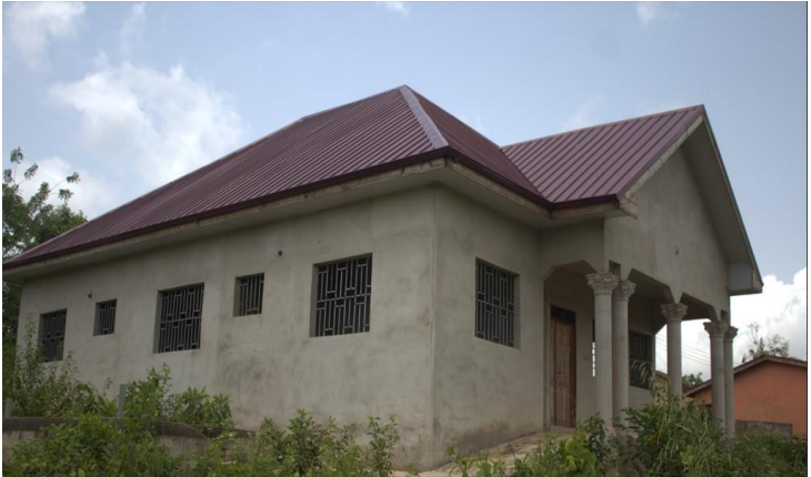
CONSTRUCTION OF CHPS COMPOUND AT DUOTU
