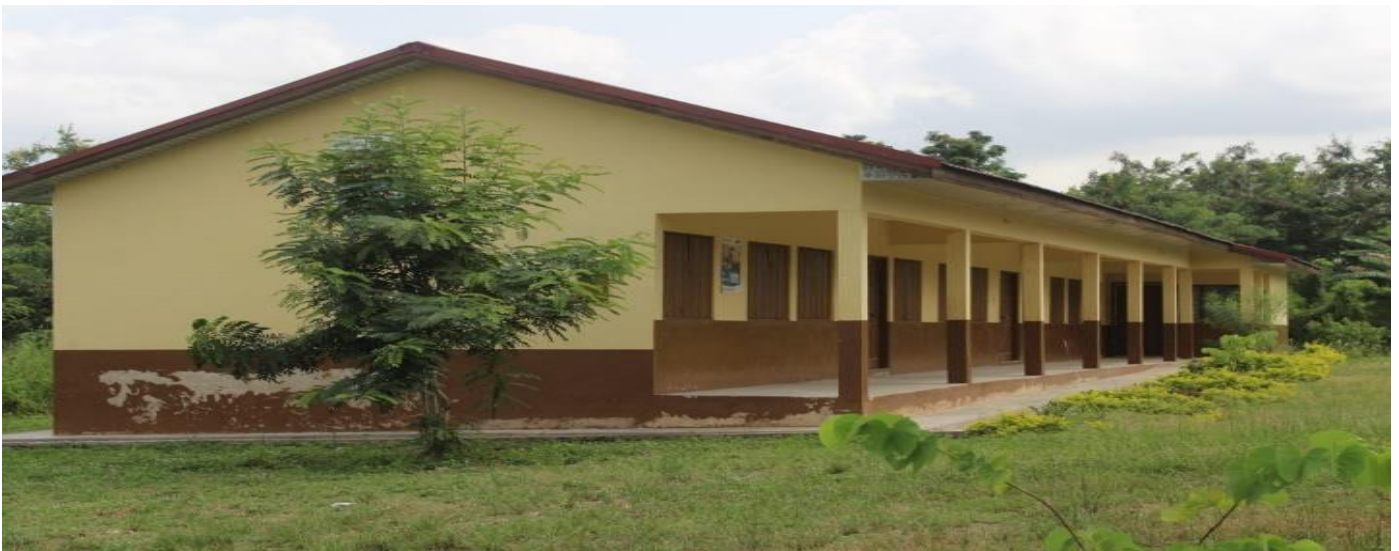
CONSTRUCTED 1 NO. 3 UNIT CLASSROOM BLOCK AT AG. TAWORA
