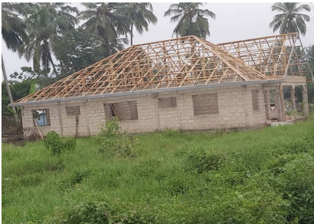
Construction of CHIP compound at Mankrong Juntion.
