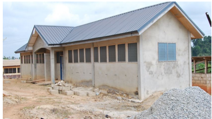
Boys Latrine at Nsaba SHS
