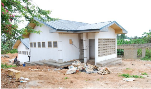
Girls Latrine at Nsaba SHS
