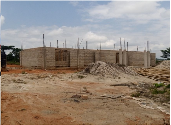
Construction of Police Station at Agona Nsaba
